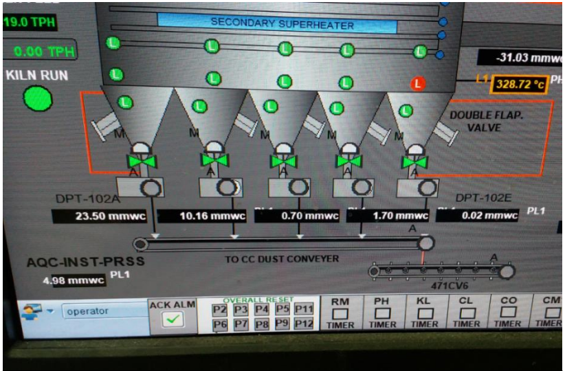
Timer based operation of AQC Boiler RAV & Chain Conveyors
